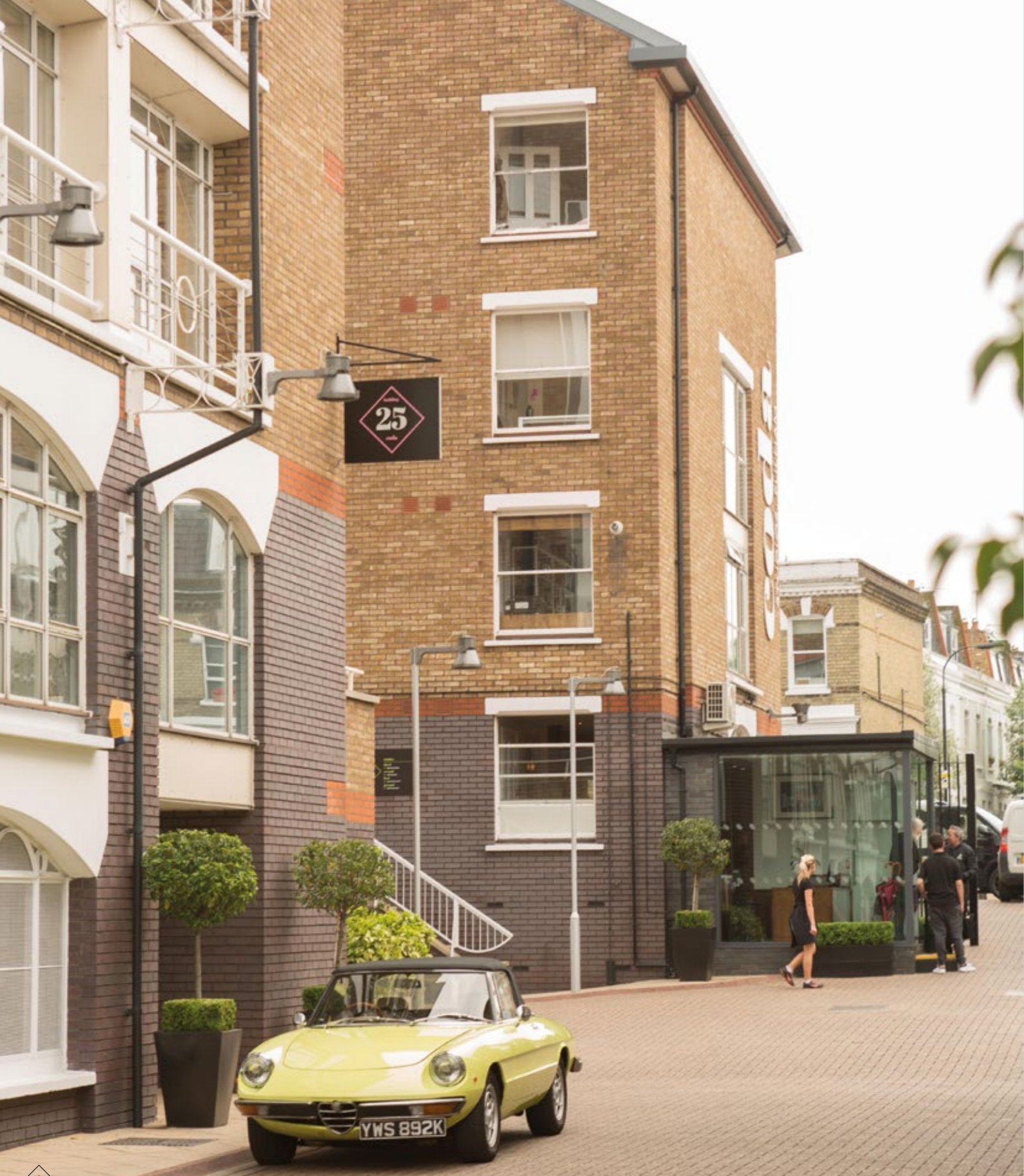
Main entrance, Coda Studios
